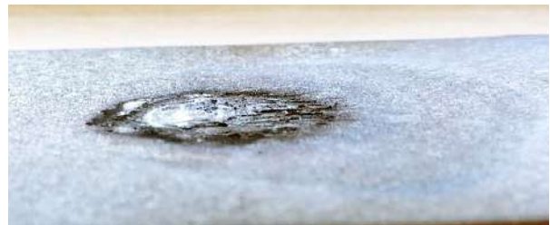
Spot weld removed
